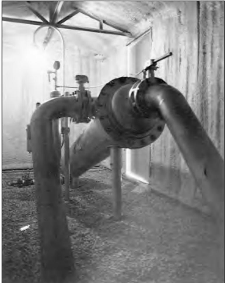
*Protected from harsh environmental elements, these Lakos "low-profile" Separators are easily enclosed in small insulated sheds or below-ground cellars.*
