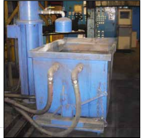
The LAKOS Separator purges into a special hopper that allows for water to rise and overflow going back to the original tank. This allows for the removal of only the scale, which sinks in the tank.
