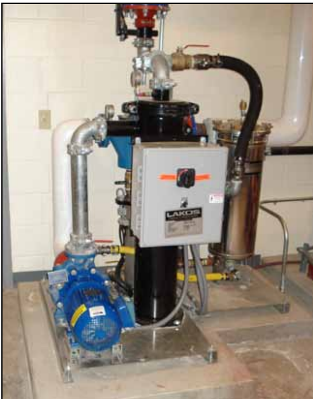
Left: LAKOS SPX-0145-SRV as a side-stream filtration unit on the Joe Crowley Student Union at UNR
