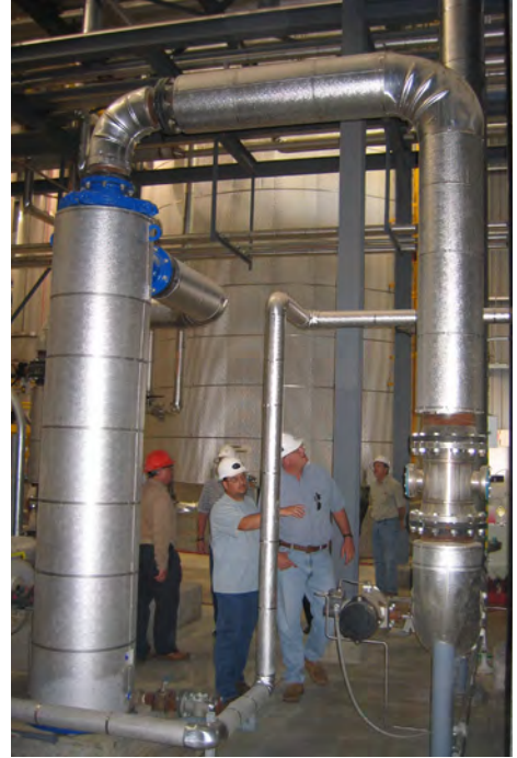
Pacific Ethanol Plant Madera, CA
