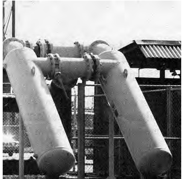
These two 12-inch Lakos Industrial Separators (above) are installed in manifold protecting one of General Electric's cooling tower systems (below, right) from troublesome and costly solids damage at their Cleveland, Ohio plant.
