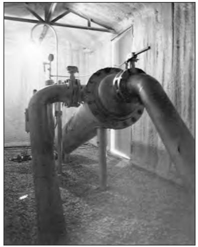
Protected from harsh environmental elements, these Lakos "lowprofile" Separators are easily enclosed in small insulated sheds or below-ground cellars.
