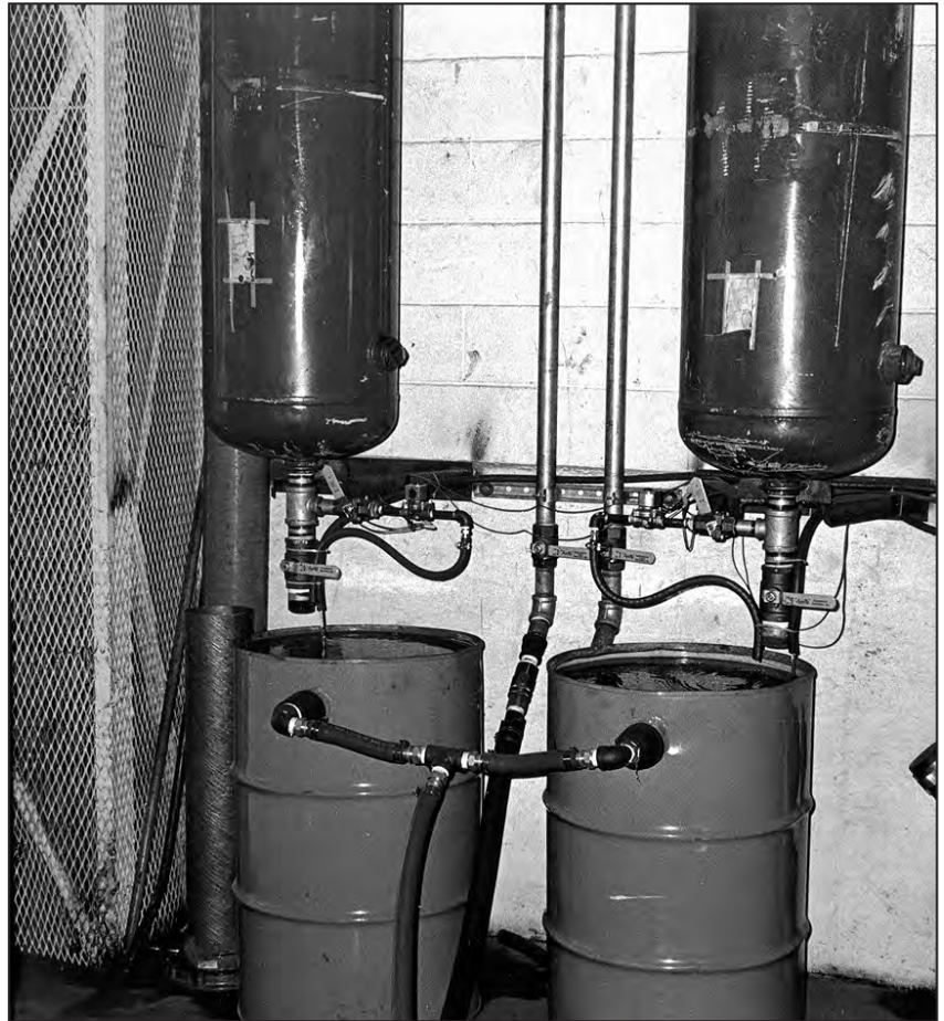
These inexpensive barrels collect the separated solids and provide an overflow for the decanted water to return to the hot well, eliminating the need for make-up water.
