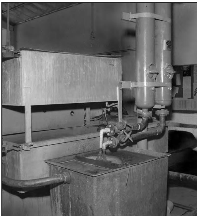
*Excess purged liquid returns to the system via an overflow hose.*
