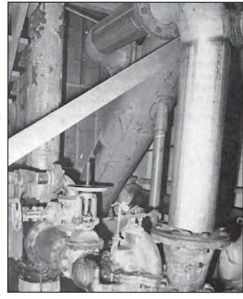
Space is limited at this paper mill. Fortunately, the Lakos Separator required very little of it to handle up to 1350 U.S. gpm (307 m3/hr) of river water for their process use.
