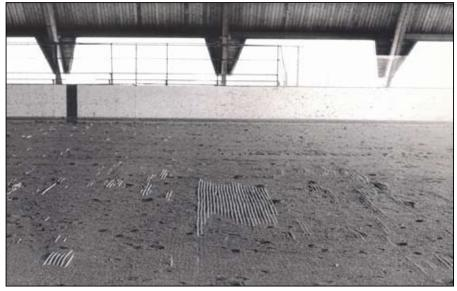
Ice rink as seen in the summer without ice. Note the extensive mat line system which covers an area in excess of 20,000 square feet (1858  $m^2$ ).
