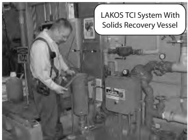
system runs continuously cleaning the cooling tower cold water basin by pulling water from the cold water basin and pumping that water through the LAKOS centrifugal action separator to remove the settleable solids. The clean water is reintroduced to the cold water basin under pressure through a piping manifold/nozzle arrangement engineered to "sweep" the basin pushing the dirt away from the cooling tower supply leaving the cooling tower and towards the LAKOS suction point.
