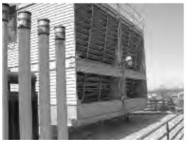
application bulletin is a single loop, primary system of two new 750 ton chillers and a 25 year old 500 ton centrifugal water cooled chiller. There are two cooling towers installed on the roof. The new approach to cooling tower basin cleaning uses a LAKOS TCI 1400 installed on the 2 cell tower.
