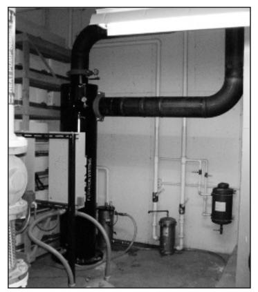
LAKOS HTH-0810 Separator installed full-stream with a Solids Recovery Vessel.
