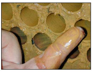
filtration in these situations is to install cooling tower basin cleaning ("sweeping") to prevent the accumulation of dirt, silt, scale and other contaminates in the system. LAKOS cooling tower basin cleaning filtration systems can remove solids from cooling tower basins down to 45 microns
