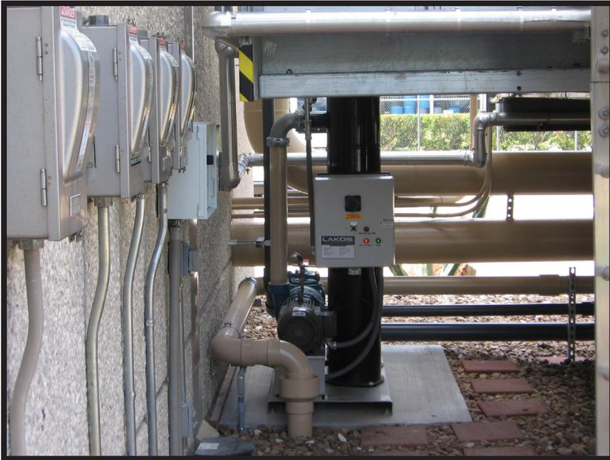
The LAKOS unit also utilizes a Solids Recovery Vessel (solids purge option) that captures solids in a sock filter allowing chemically treated and filtered water to be reintroduced to the system loop. This solution allows the Texas laboratory to tout a zero liquid loss approach to filtration.
