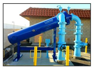
**Solution:** The district's engineering group recommended two LAKOS JPX Sand Separators, because of their fine sand removal performance (200 mesh/74 microns) and their ability to be automated. The LAKOS solution also meant eliminating routine maintenance, and no cleanable or replaceable filter elements. A LAKOS Separator also meant an even, lower pressure loss, enabling the water treatment systems to see a steady flow and pressure for optimum performance.
