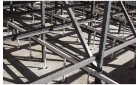
HydroBooster layout in field erected cooling tower
