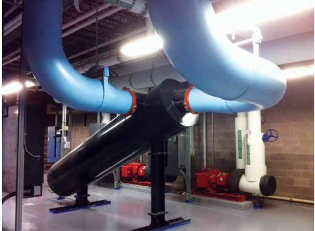
LAKOS HTH 3500 used to keep wind-blown sand from damaging heat exchangers and other equipment in manufacturing plant in New Mexico.
