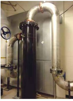
HTX installed at Peppermill Casino in Reno, Nevada, keeps their geothermal heat exchanger clean and free of dirt. The Peppermill has won numerous awards for its facility, including Green Company of the Year
