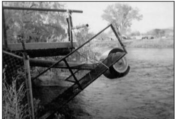
Pumping 640 U.S. gpm (145 m<sup>3</sup>/hr) at 90 psi (630 kPa), this pump station in Wyoming relies on a PLUM CREEK Screen to prevent organics and debris from interrupting water service to its customers. A galvanized steel shield has been added for protection against large or heavy objects carried by the river's swift current. Note the shield's notched side-opening that allows PLUM CREEK's backwash jets to blow away particles attracted to the screen.
