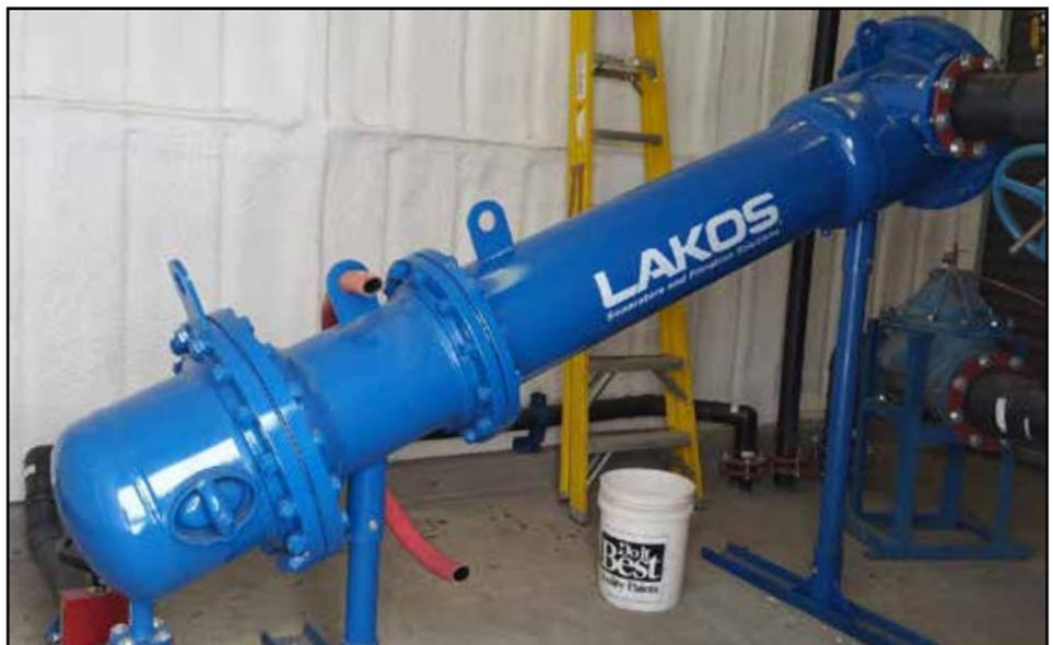
JPX-0650-L/FLG/EC/NS separator was designed specifically for this application.
