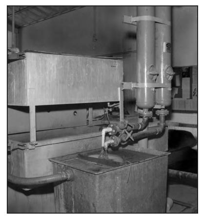
Excess purged liquid returns to the system via an overflow hose.
