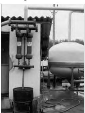
to plant use. The purging of solids from the separators is accomplished via continuous bleed into a drum, allowing excess liquid to decant for easy solids handling.
