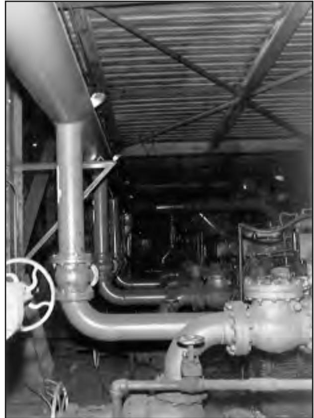
*From the main discharge line of the LAKOS Separators, as many as five high pressure pumps draw solids-free water to feed high pressure nozzles. This protects both the pumps and nozzles from excessive wear.*
