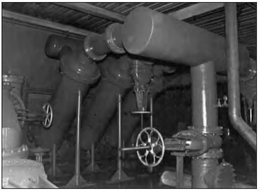
Nicknamed the "Blue Goose," this LAKOS manifold system handles up to 18,000 U.S. gpm (4,088 m<sup>3</sup>/hr). Separated solids are bled continuously into an open trough via a manual pinch valve. Plans are scheduled, however, to install LAKOS heavy-duty bleed-purge hardware.
