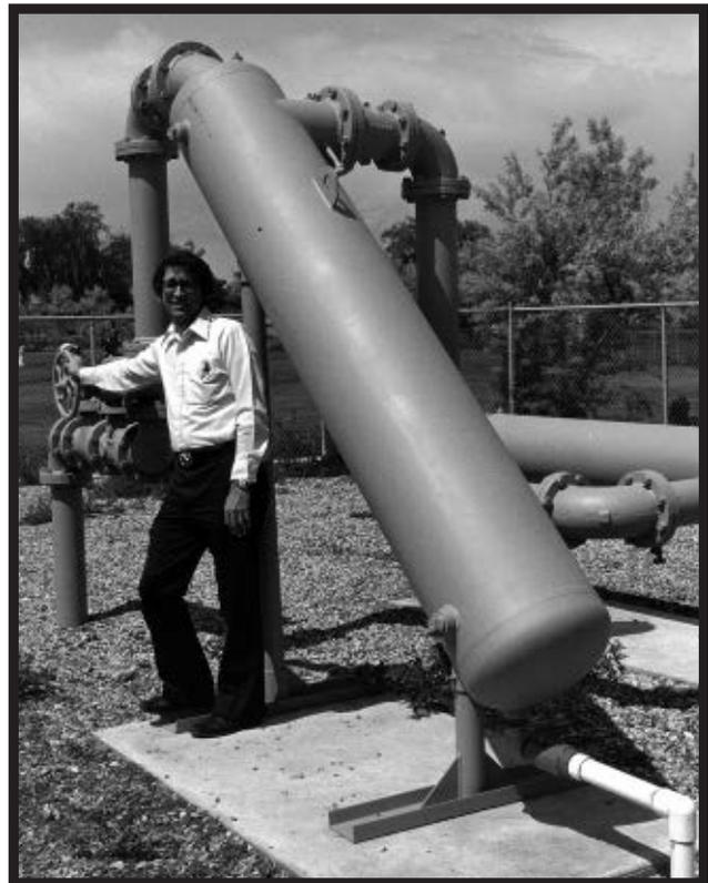
Carl R. Nelson, Jr. stands beside Lakos Separator installation at Mick Riley Golf Course, Salt Lake City. Drawn from lakes, water is pumped through screen and Lakos unit to sprinkler system.
