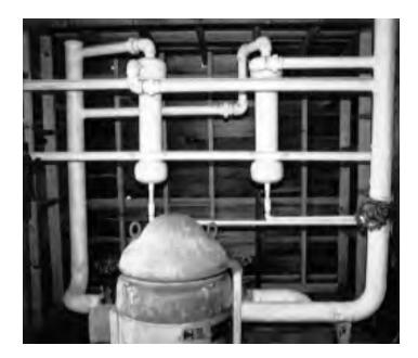
In addition to the increased labor/maintenance costs, the sand-clogged valves subsequently allowed hard water to enter the boiler, resulting in a buildup of scale.
