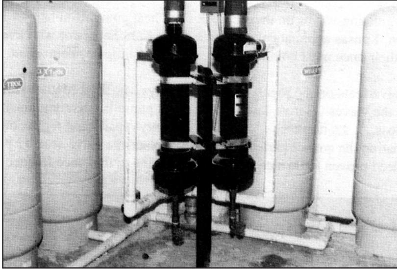
*This pair of LAKOS Separators, installed by Price Water Well Service at a state government facility in Hutchinson, Kansas, protects a system of 13 heat pumps from a serious problem of troublesome sand and grit. “Without the separators, “ says Mattison, “we would have had to replace more than two dozen valve seats in the regulating valves at a cost of almost \$1,000.”*
