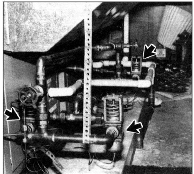
*Installed nearly against a wall near the pressure tank and water conditioning equipment (photo at left), this LAKOS Separator provides sure protection for a heat pump system's regulating valves (right). Close quarters and the typical maze of plumbing for such installations further underscores the value of LAKOS Separators to help eliminate valve and maintenance problems.*
