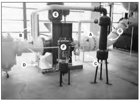
scale deposits are then collected into a Lakos Closed Recovery System (CRS), allowing excess purged water to flow back into the HVAC system and eliminating water waste and water treatment chemical waste.
