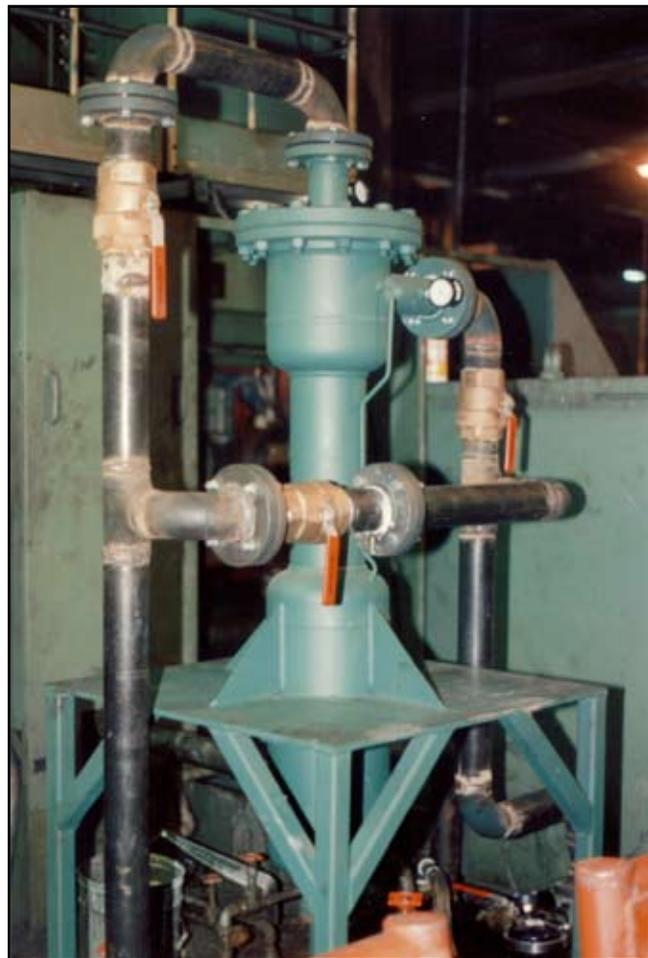
*Lakos AXL Series Separator filtering solids from Southwire's 170 U.S. gpm, full-stream quench oil supply line.*
