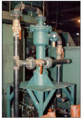
Lakos AXL Series Separator filtering solids from Southwire's 170 U.S. gpm, full-stream quench oil supply line.
