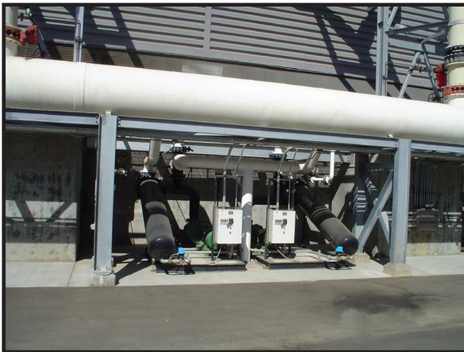
The medical center's central utility plant is an 11,000 ton system with multiple absorption and centrifugal electric chillers. To allow for continuous operation during the new system construction, the new cooling towers were located next to the existing towers. Plant operators noted that the existing condenser water system had been a trouble spot almost since the startup of the original system.
