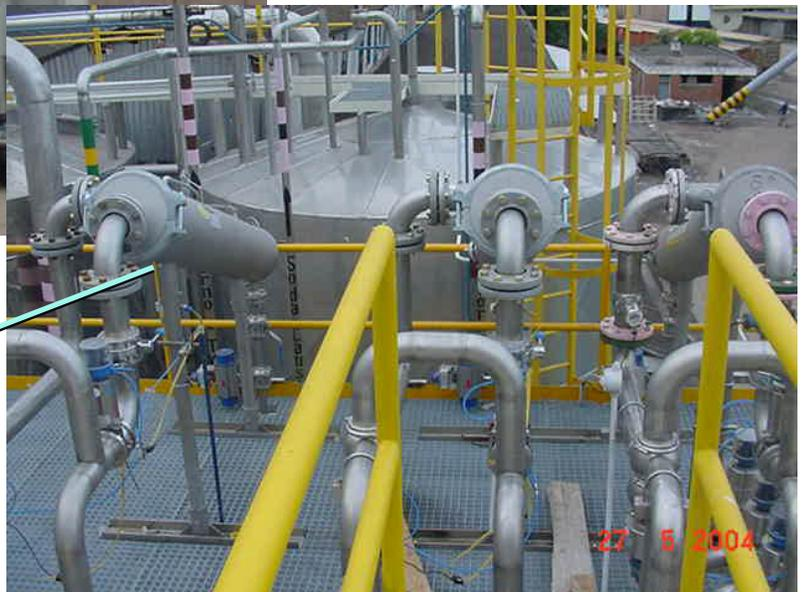
LAKOS Stainless Steel Separators help to keep unwanted solids from clogging CIP Systems. The need for continuous operation (with little or no downtime) is critical for CIP operating efficiency ... and LAKOS Separators meet that need with continuous operation, automatic solids flushing, and a low and steady pressure loss.
