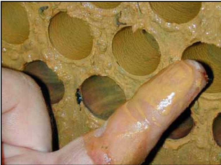
filtration in these situations is to install cooling tower basin cleaning (“sweeping”) to prevent the accumulation of dirt, silt, scale and other contaminants in the system. LAKOS cooling tower basin cleaning filtration systems can remove solids from cooling tower basins down to 45 microns.
