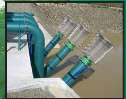
Rotating Screen Reduces Clogging
