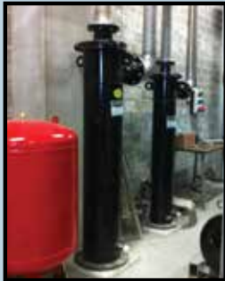
Cleaning chilled water, Axima Belgium
