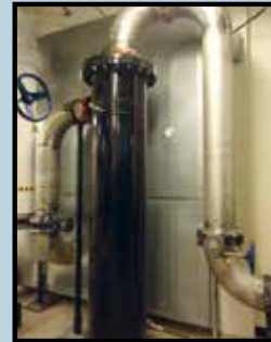
Protecting heat exchangers, Nevada USA
