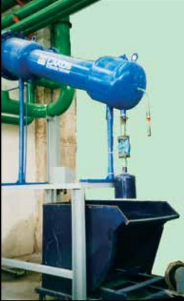
After the solids are removed from the process flow, LAKOS offers several manual or automatic SOLIDS HANDLING purge options to capture and concentrate the solids for disposal at low cost and low maintenance. These include everything from simple barrels and collection hoppers to automated valve options as shown.
