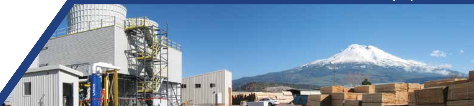
Prevent Solids Accumulation in Sumps and Basins
