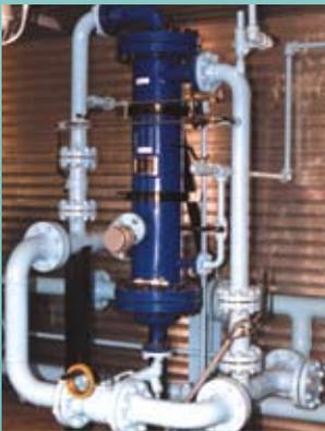
▶ **A waterflood injection site** depends on a LAKOS Desander to extend the life of its oil/water hydrocyclone by removing abrasive particles. This LAKOS 740 psi (51 bar) system replaced a bag filter with greater efficiency, lower pressure loss and reduced maintenance requirements.
