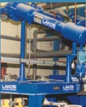
▶ **Sandy river water** is pre-filtered with a LAKOS Desander to protect ultrafiltration equipment from excessive maintenance routines prior to high pressure injection wells.
