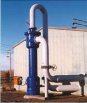
▶ **As primary filtration,** a LAKOS Desander keeps sand & silt from river water out of a plant's piping system, reducing overall system maintenance and fouling.
