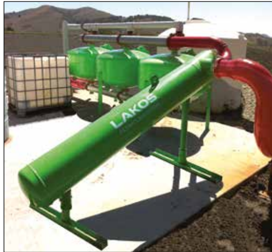
BRS- Backwash Reduction System
